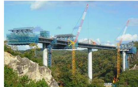
**Photo 3** Cantilever erection
