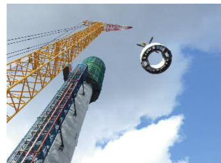
Photo 2 Installing half-precast components
